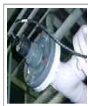
Remote Sensor Flanged Adapter 150# RF flange fitting for toxic sensors
